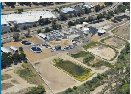
The City of Paso Robles operates a 4.9 mgd activated sludge wastewater treatment plant (WWTP) to meet the needs of 36,000 plus residents and a number of local vineyards and wineries. Treated wastewater from the facility is used for GWR to replenish the Paso Robes water basin and Salinas River. The facility faces stringent NPDES permit restrictions on effluent levels of total nitrogen (TN), microbiology and THMs.
